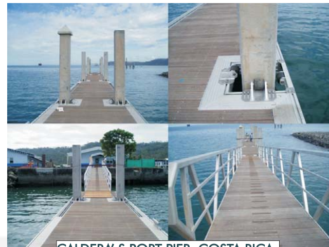
CALDERA' S PORT PIER. COSTA RICA.
